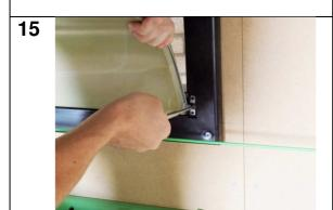
Slide the flap simultaneously into the housing.
