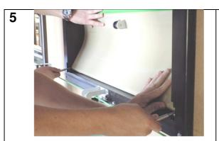
Remove the flap with two persons at the same time by holding the flap firmly and pull back the spring tool. Carefully loose tension of the springs.
