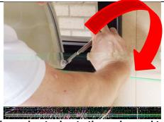
Put the spring tool onto the spring and turn it ¾ stroke backwards. Do this with two persons on both sides at once. Hold the flap firmly tight!
