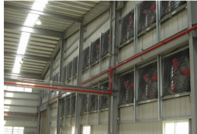
Ventilation in factories in Asia
